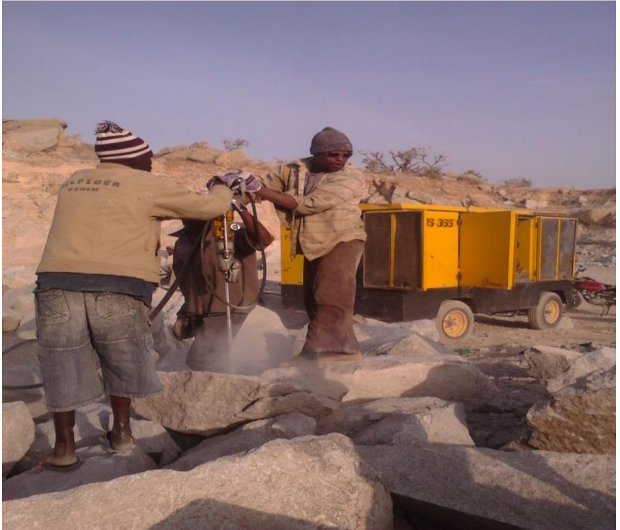
Figure 8: Handheld Drill (Jackhammer) Machine for Secondary Blasting
