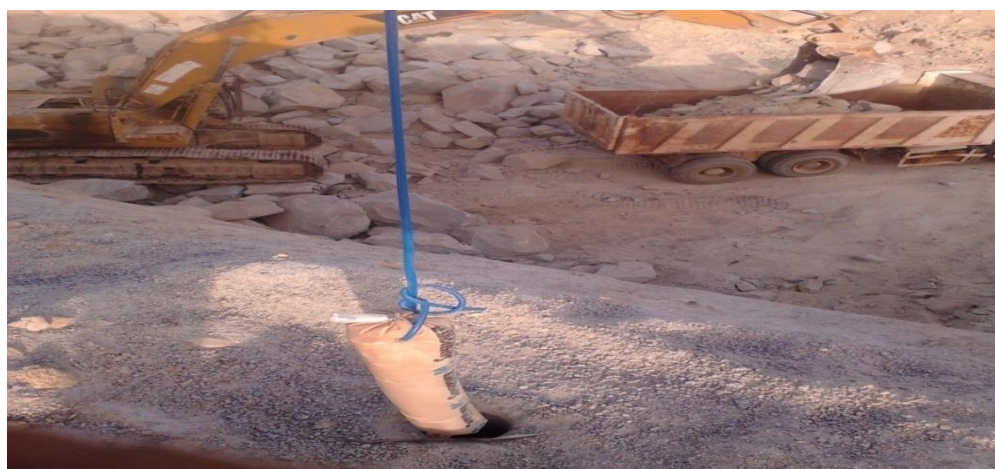
Figure 7: Priming of Holes for Primary Blasting
