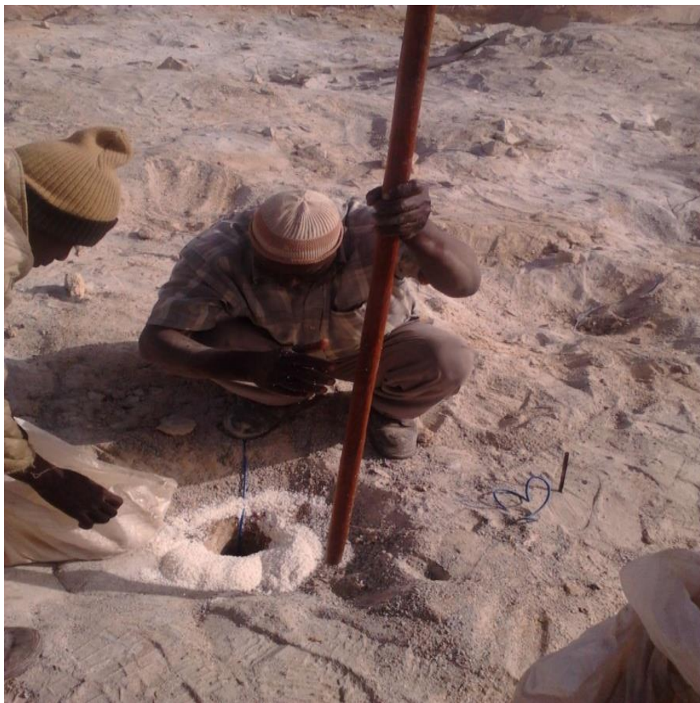
Figure 6: Charging of Holes for Primary Blasting
